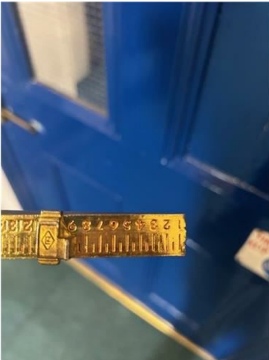
Hazel Main excessive door gap 5.jpg
