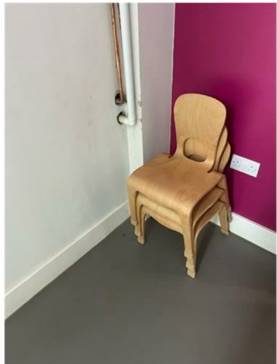
Hazel Bailey Combustible chairs in protected staircase 2.jpg
