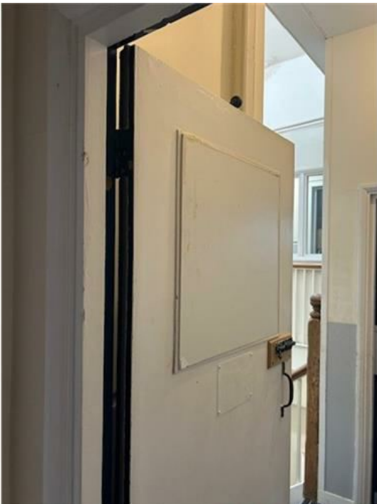
Hazel Main FD onto protected staircase.jpg
