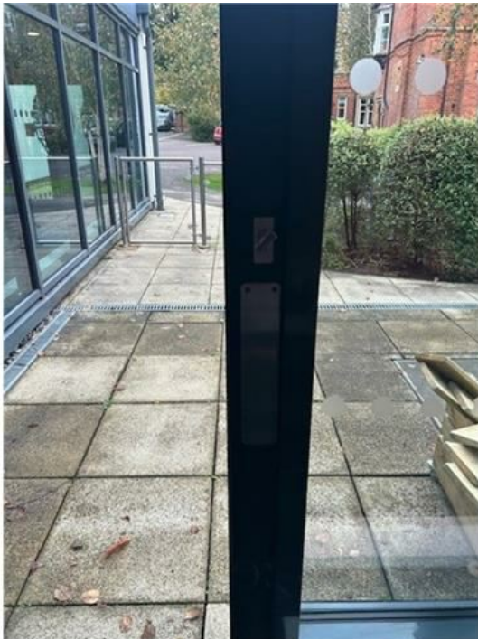
Hazel Bailey No sign for opening device.jpg
