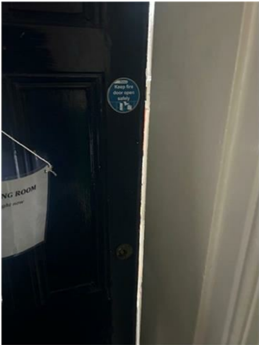
Hazel Main excessive door gap SEND 3.jpg
