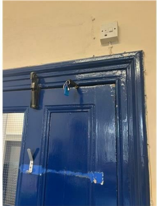
Hazel Main excessive door gap 6.jpg
