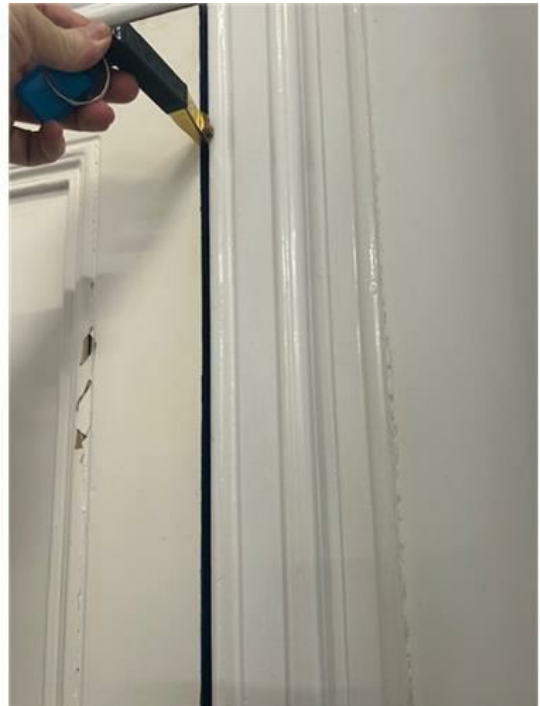
Hazel Main excessive door gap 6.jpg
