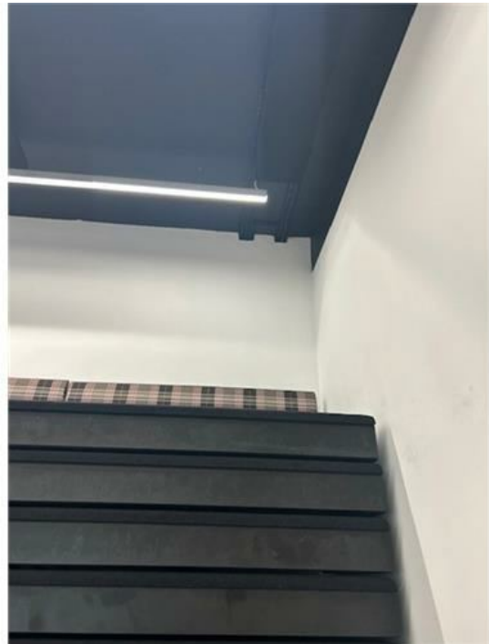
Hazel Bailey Holes in Bawtree wall 2.jpg
