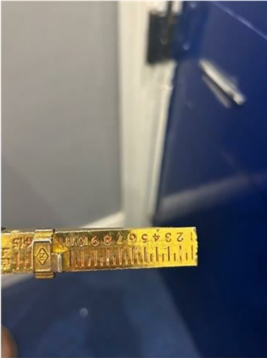
Hazel Main excessive door gap 5.jpg
