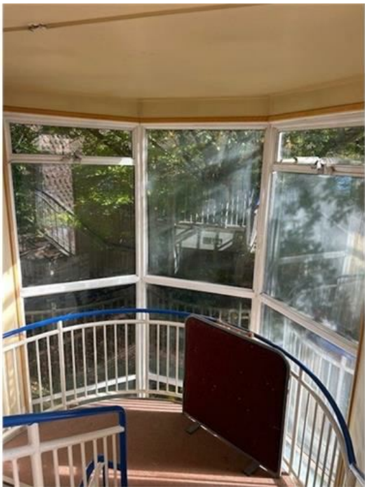
Hazel Meadow combustibles in protected staircase 2.jpg
