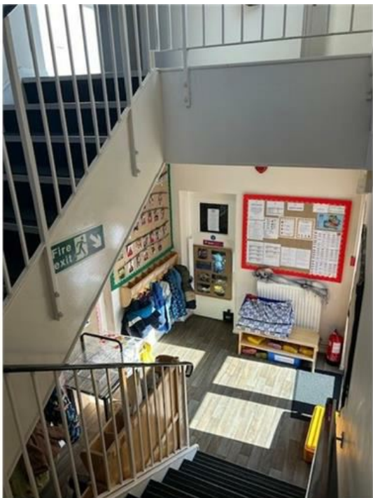
Hazel Meadow combustibles in protected staircase 2.jpg
