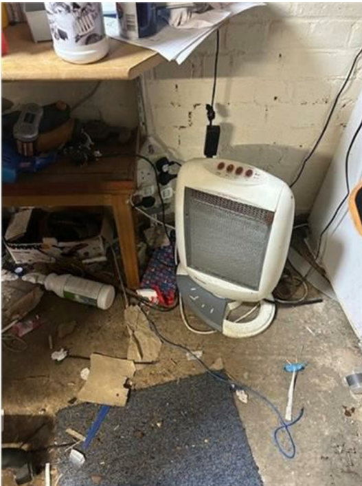
Hazel Orchard overloading of adapter.jpg
