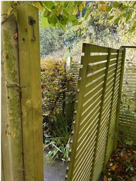
Hazel Elm Escape route gate replaced.jpg
