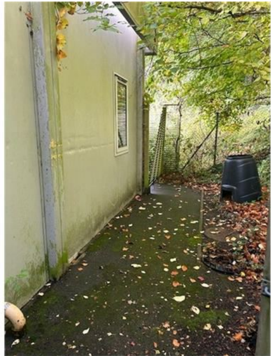
Hazel Elm Escape route gate replaced 2.jpg
