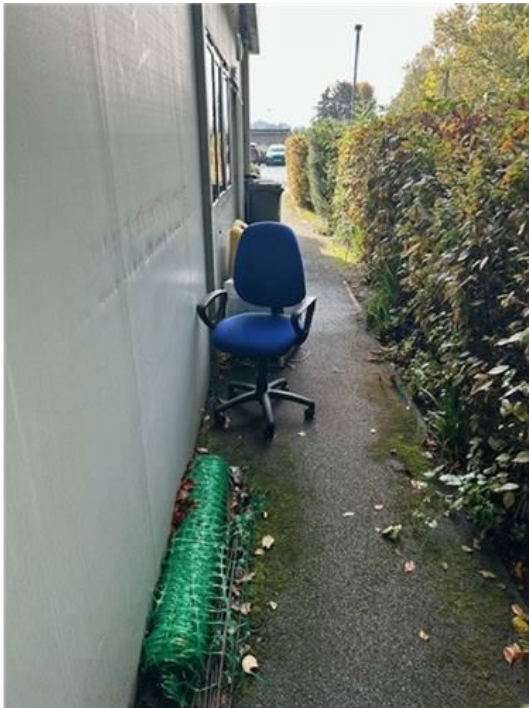
Hazel Elm Escape route obstructed.jpg
